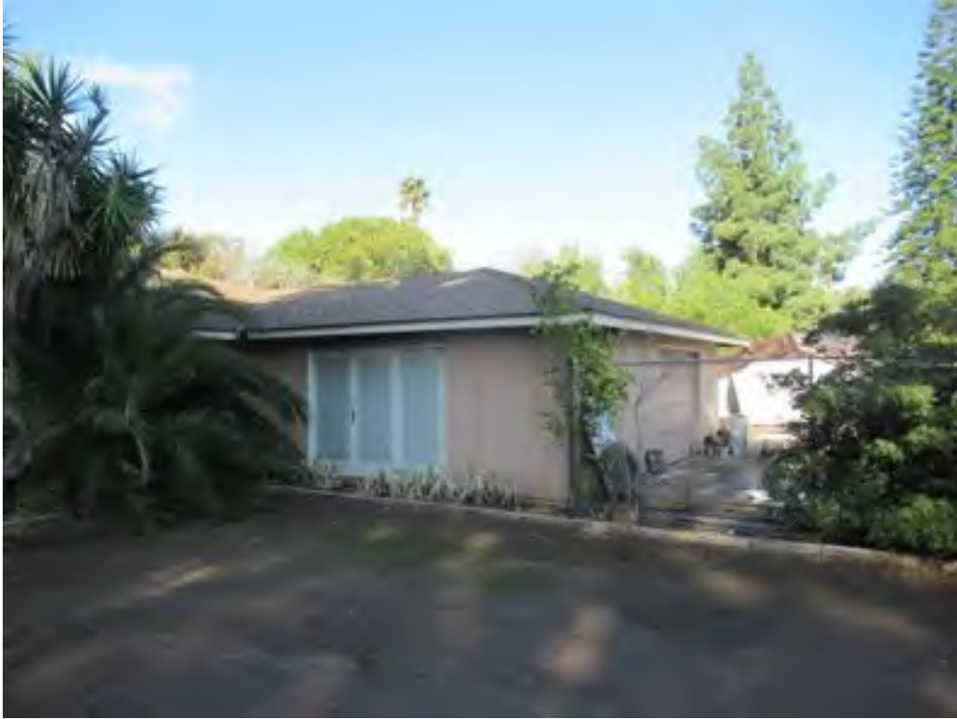
77. Typical building exteriors at 18602 Altrudy Lane.
