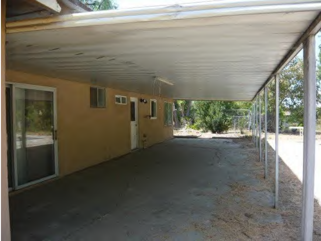
29. Typical building exteriors at 18602 Altrudy Lane.
