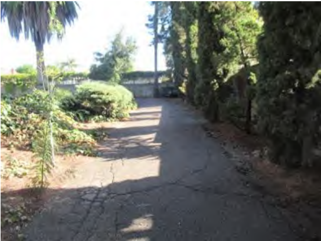
2. Typical asphalt-paved drive area.
