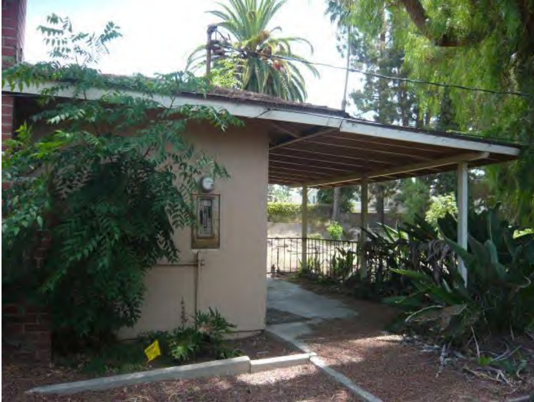
25. Typical building exteriors at 18602 Altrudy Lane.
