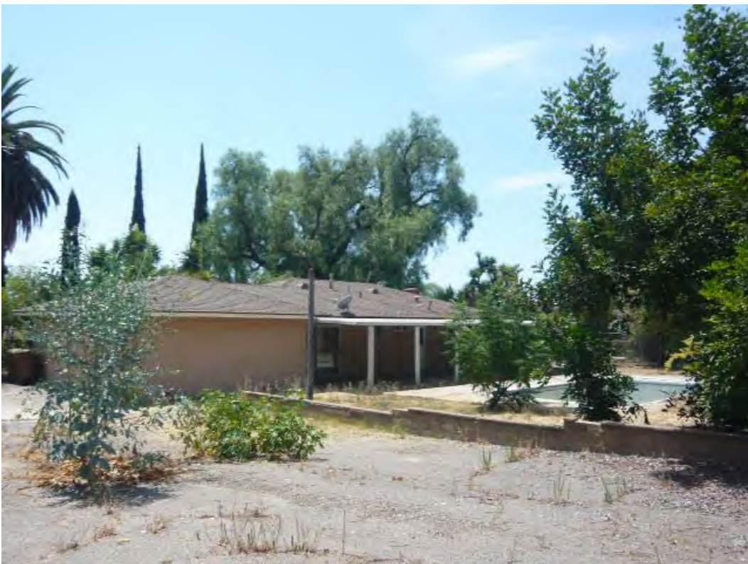
24. Typical building exteriors at 18602 Altrudy Lane.
