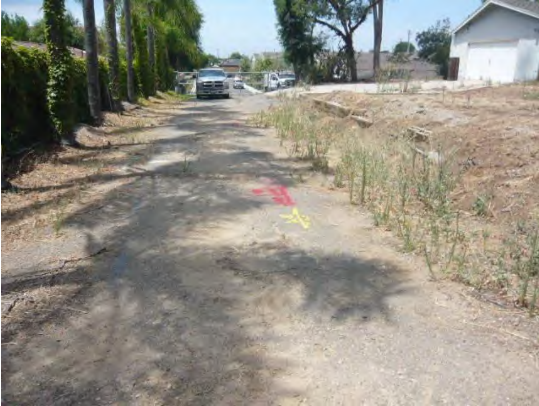
1. Typical asphalt-paved drive area.
