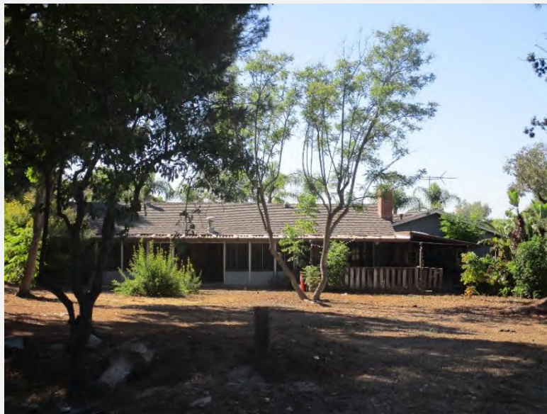
Photograph 2. Rear (north) elevation of the residence at 18597 Altrudy Lane, view looking south. Photograph taken on October 22, 2024.
