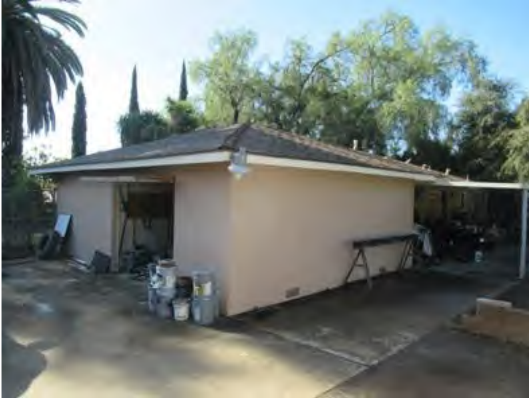
79. Typical building exteriors at 18602 Altrudy Lane.
