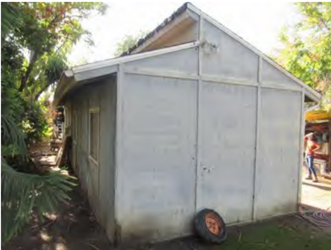
52. Storage building at 18597 Altrudy Lane.
