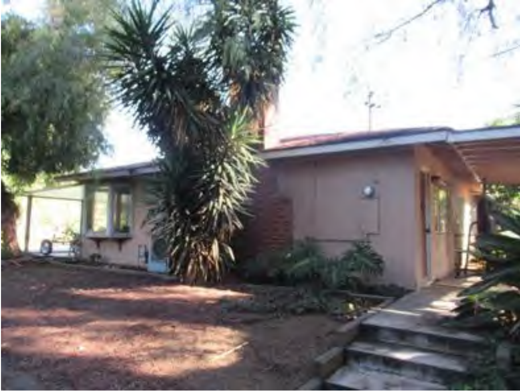
75. Typical building exteriors at 18602 Altrudy Lane.
