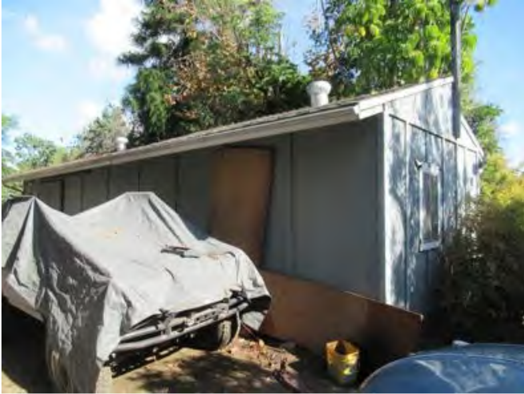
51. Storage building at 18597 Altrudy Lane.
