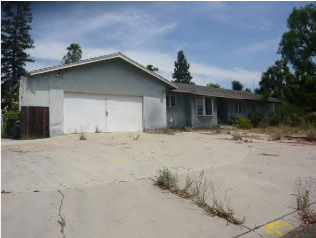
8. Typical building exteriors at 18597 Altrudy Lane.
