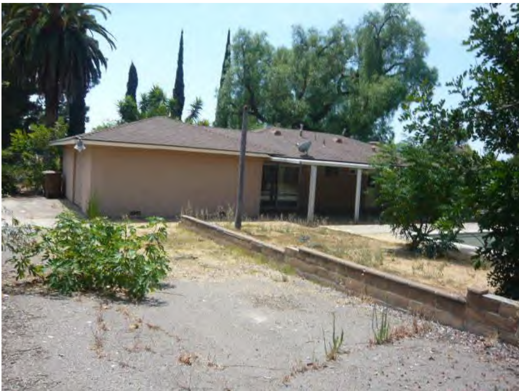
28. Typical building exteriors at 18602 Altrudy Lane.
