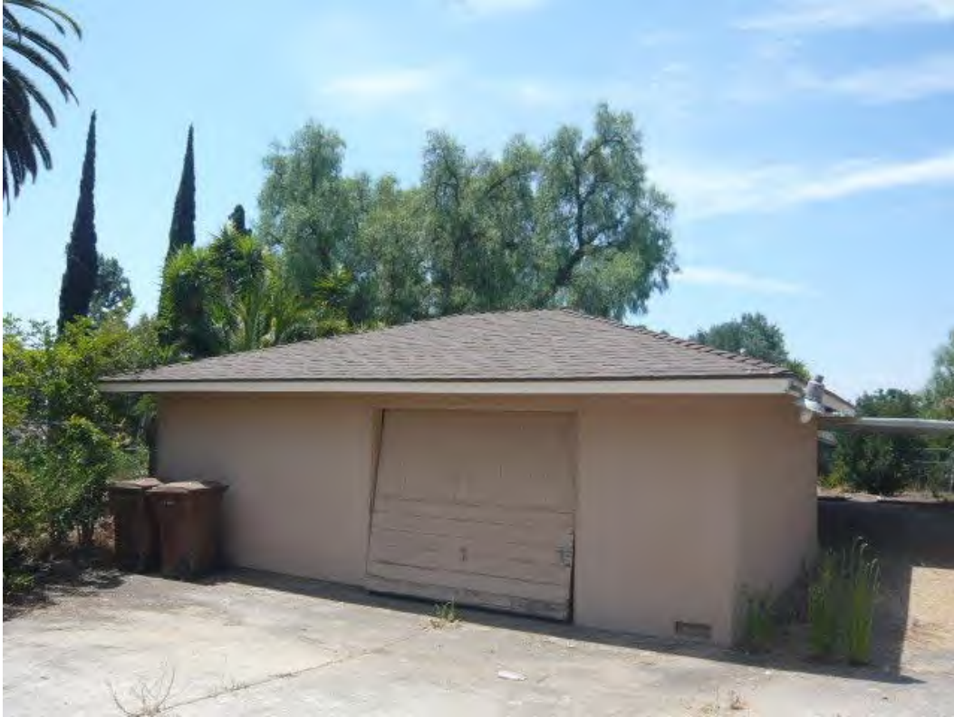
27. Typical building exteriors at 18602 Altrudy Lane.
