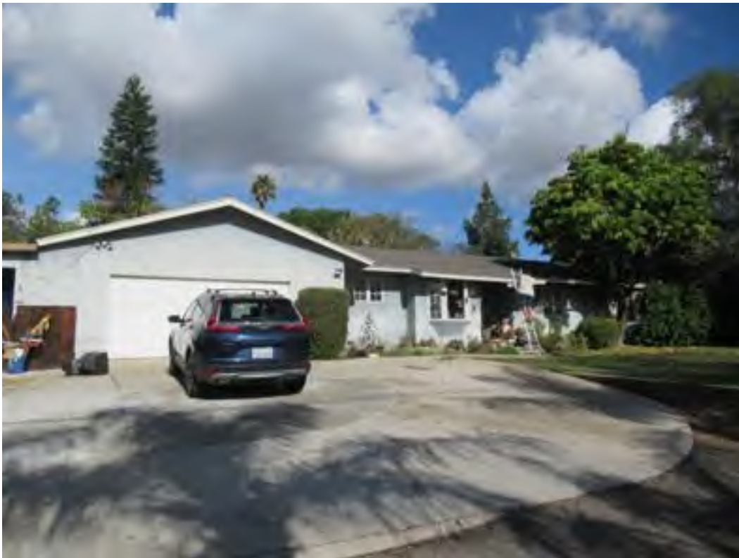
30. Typical building exteriors at 18597 Altrudy Lane.
