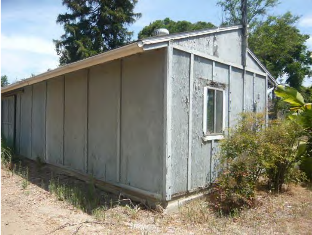
15. Storage building at 18597 Altrudy Lane.
