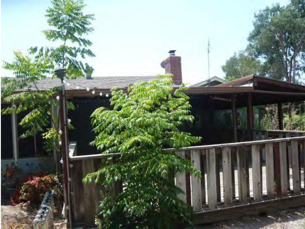
11. Typical building exteriors at 18597 Altrudy Lane.
