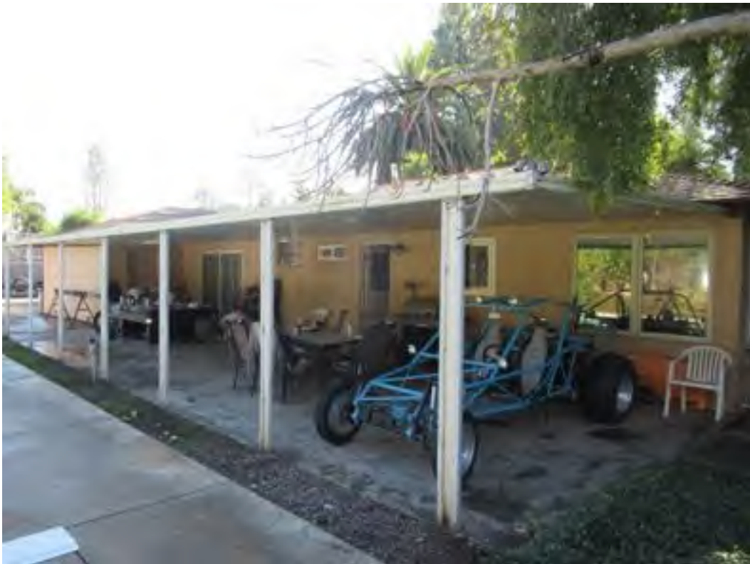
78. Typical building exteriors at 18602 Altrudy Lane.
