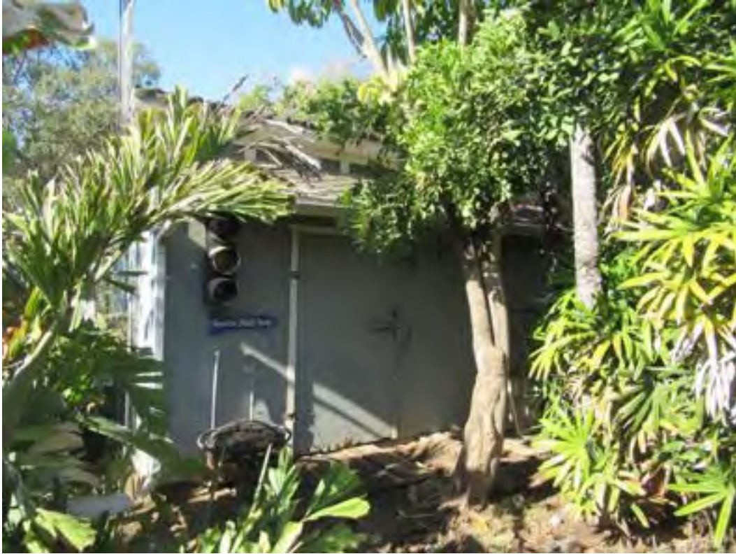
53. Storage building at 18597 Altrudy Lane.
