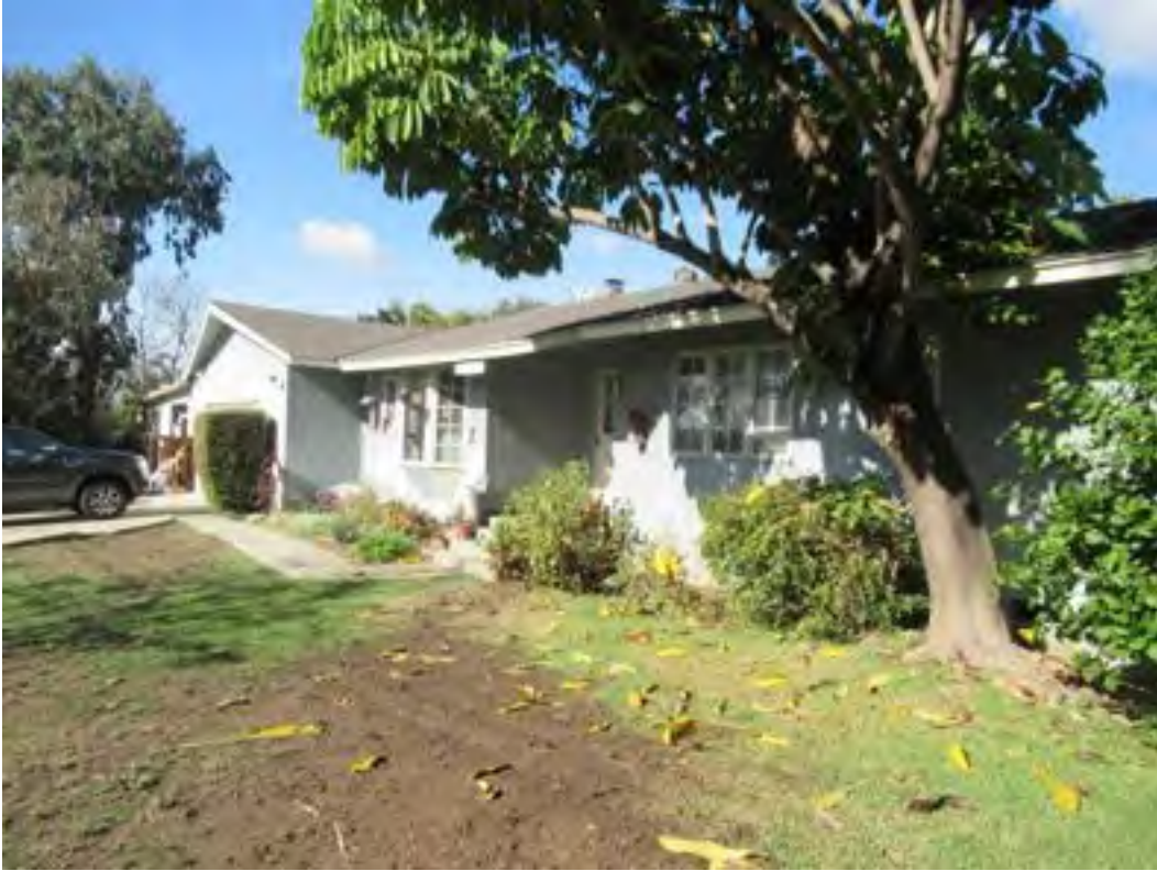
31. Typical building exteriors at 18597 Altrudy Lane.
