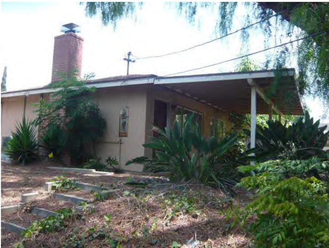
26. Typical building exteriors at 18602 Altrudy Lane.
