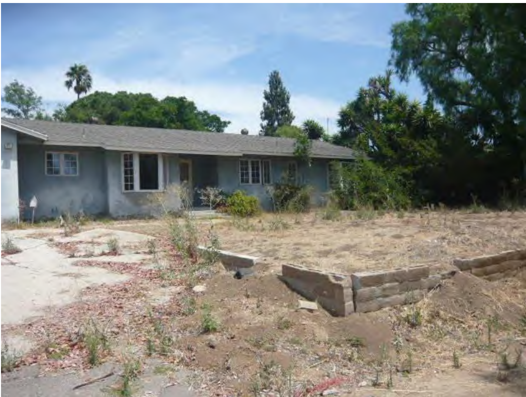
2. Landscaping and septic tank area at 18597 Altrudy Lane.
