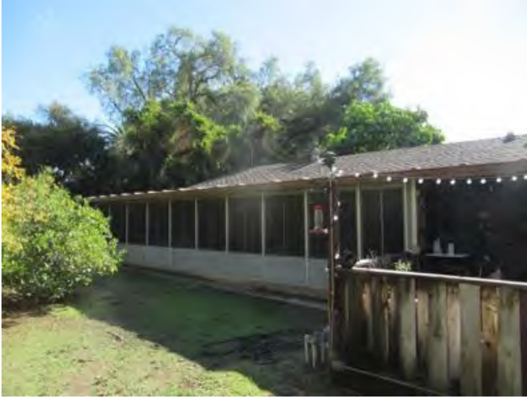
33. Typical building exteriors at 18597 Altrudy Lane.
