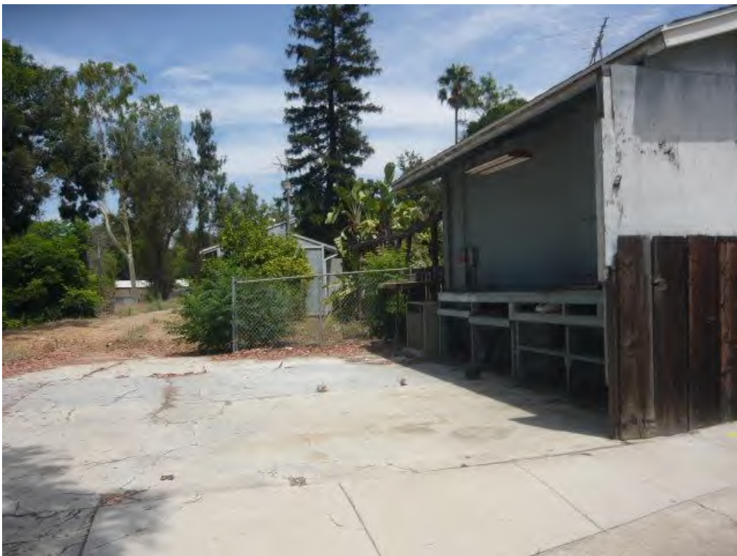
12. Typical building exteriors at 18597 Altrudy Lane.
