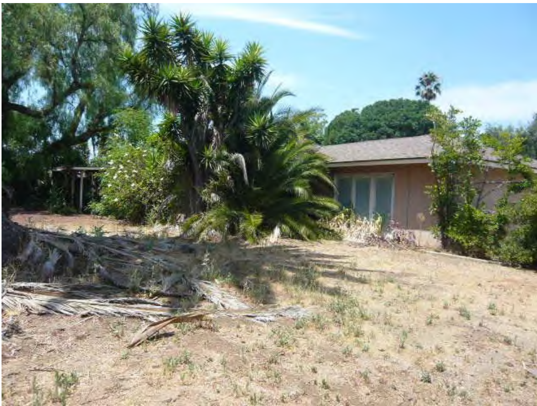
30. Typical building exteriors at 18602 Altrudy Lane.
