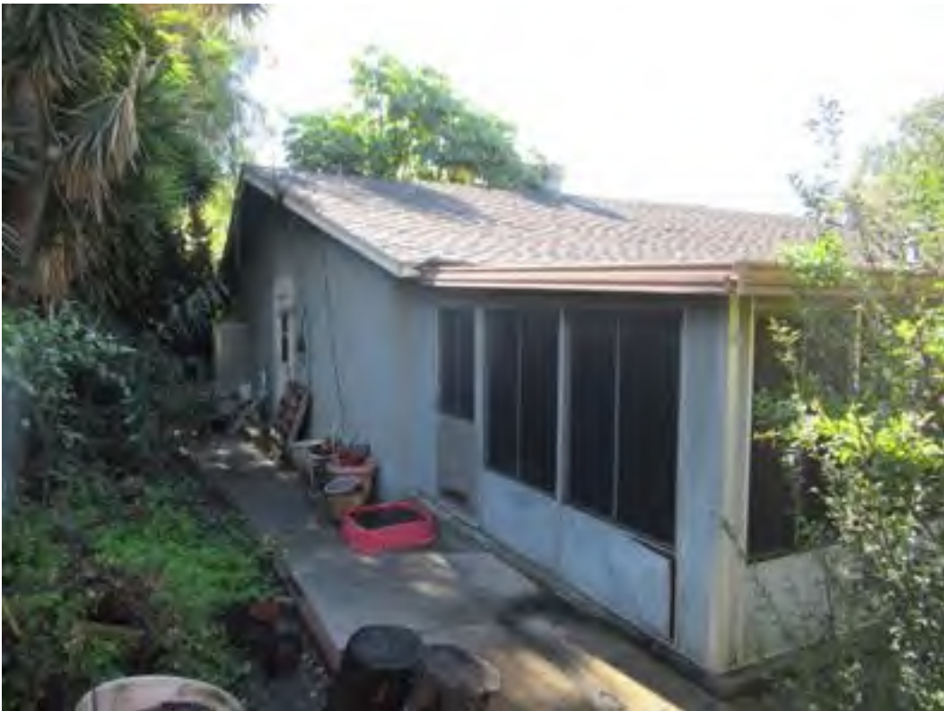
32. Typical building exteriors at 18597 Altrudy Lane.
