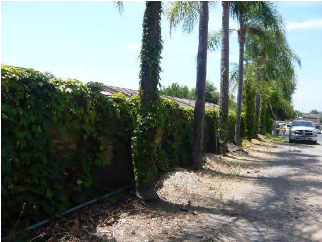
36. Lakeview Townhomes (multi-family residential) adjacent to the south of the subject property.
