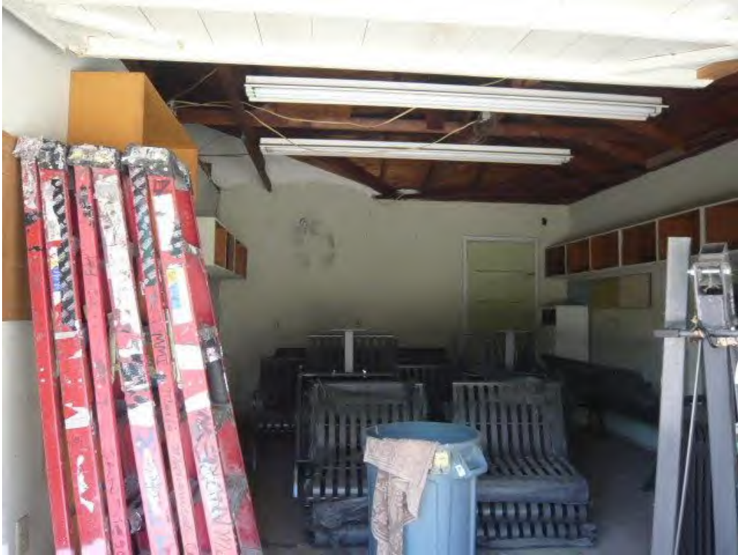
31. Typical interiors at the garage at 18602 Altrudy Lane.
