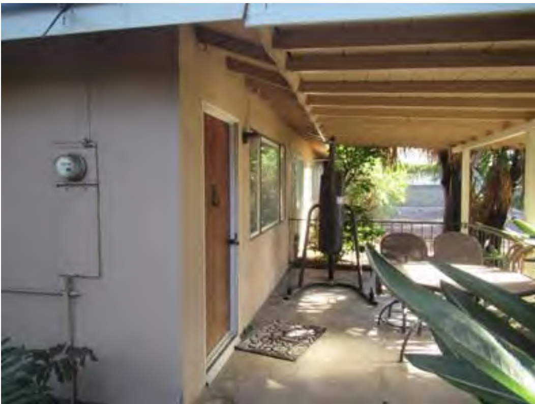
76. Typical building exteriors at 18602 Altrudy Lane.
