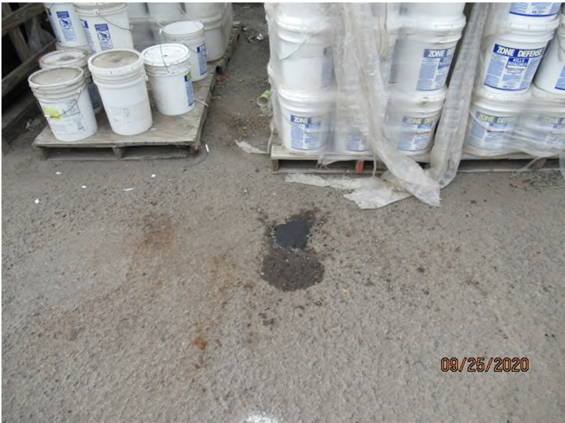
Photo 2 - The cement patch, dyed black, is shown for soil boring SB-9. A similar patch was placed for soil boring SB-8, located west of the buckets of orthoboric acid.
