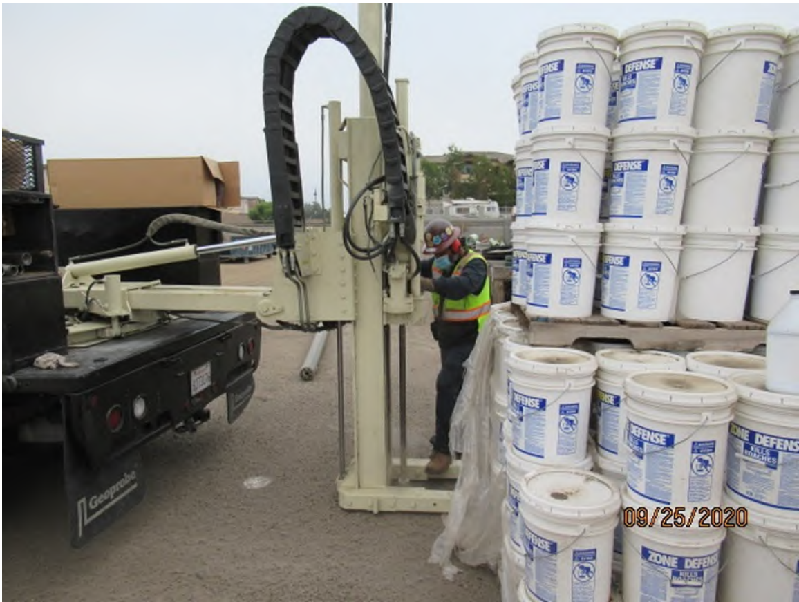
Photo 1 - View facing east, showing the Interphase Environmental, Inc. direct-push rig breaking through the asphalt at soil boring SB-9, prior to hand auger advancement of the soil boring for soil sample collection to assess potential impacts from the buckets of orthoboric acid shown to the right.
