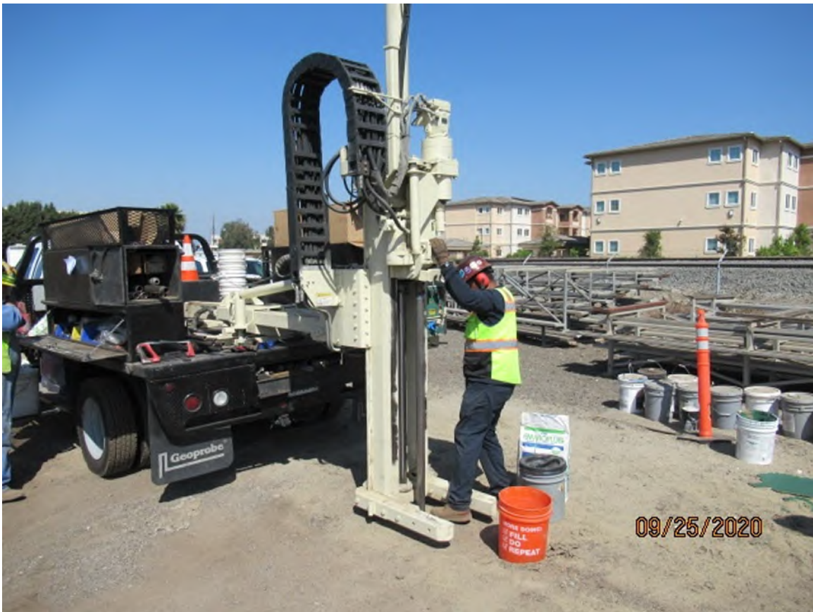
Photo 3 - View facing northeast, showing the direct-push rig advancement at SB-3/SVP-3. Construction materials for the soil vapor probe are shown near the advancing push rod, including bentonite granules, #3 Monterey sand, and water.
